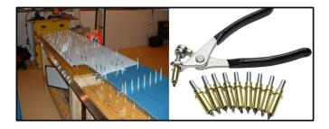
The Elevator build sequence is tedious: Clecos (right) are used to hold parts together for fabrication. Lots of holes are drilled, fitting, redrilling, and finally rivets. **Extra Eyes:** Building comes with challenges. Sometimes the instructions are ambiguous, parts do not seem to fit like I think they should, or the there is a single step in the build manual that says, "Install everything forward of the firewall."
